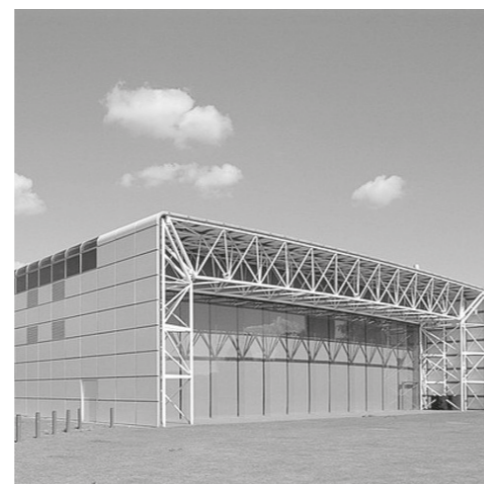
Sainsbury Centre of Visual Arts Foster + Partners
